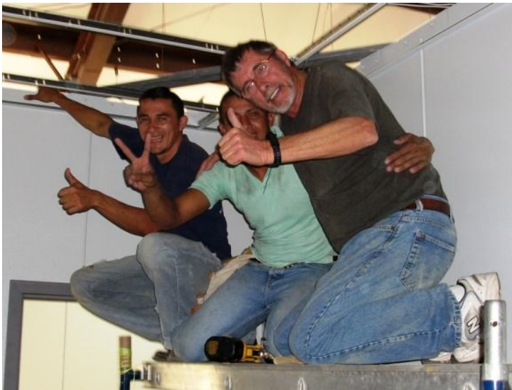
Jack Williams & Crew placing T-Bar Ceiling
