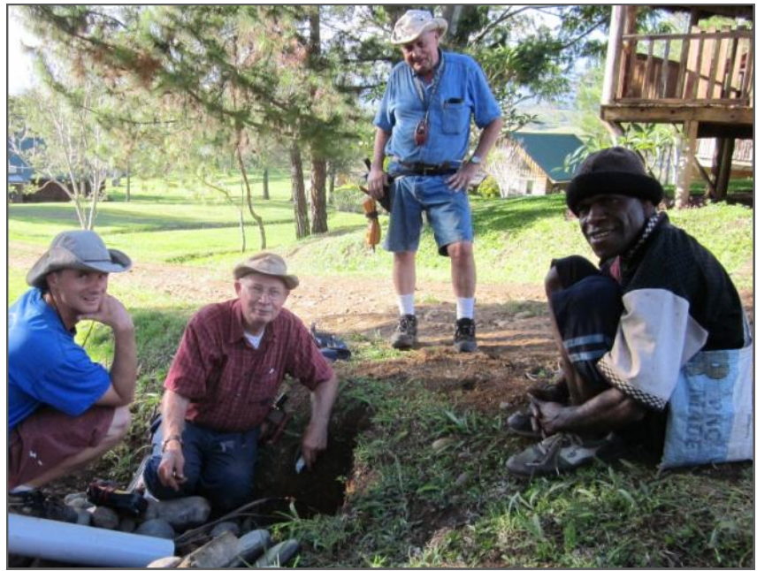
Missionary Jacob, Earl, Jerry and Michael repairing a cable
